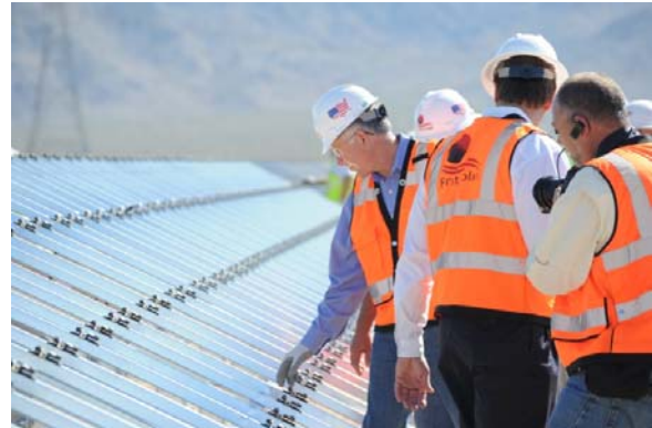
Secretary Salazar examines a solar energy project under construction on public lands in Nevada
