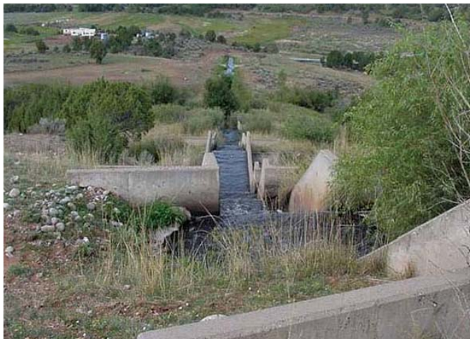
Drop Structure – Pine River Irrigation Project
