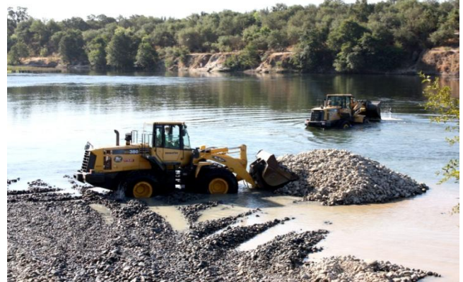
Spawning gravel being placed in the Lower American River
