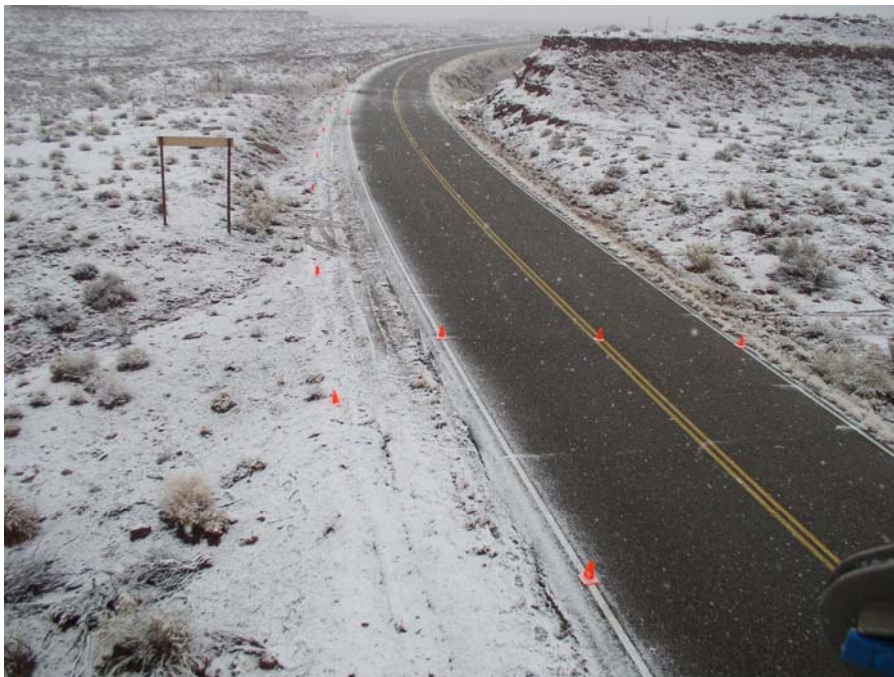
Figure 3. Tire marks on roadway (row of traffic cones to left of roadway follow the tire marks onto the foreslope).
