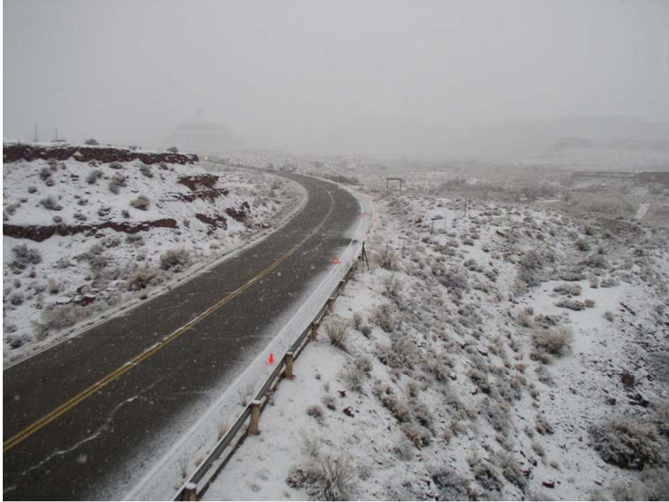
Figure 11. View of descending road grade in the direction of travel, immediately preceding the accident curve.
