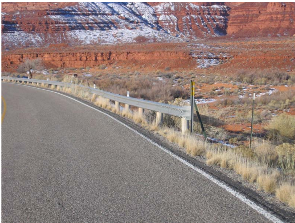
Figure 13. View of guardrail.
