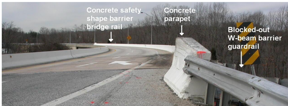
Figure 5. I-895 overpass barrier system.
