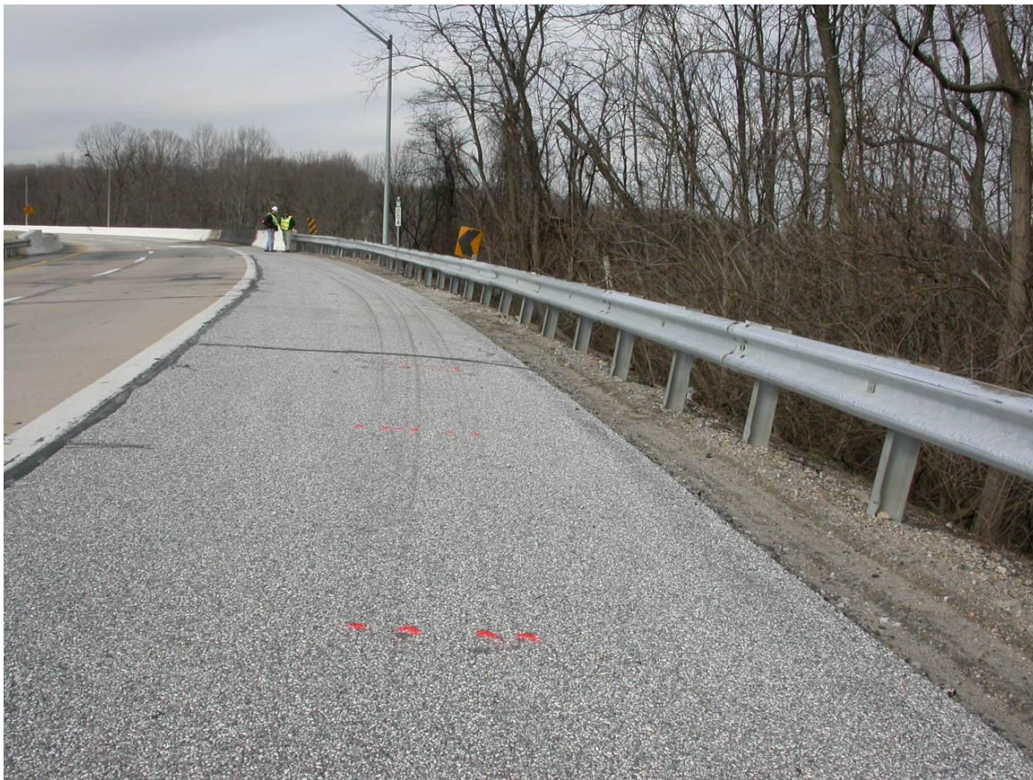
Figure 2. View of tire scuff marks leading to the overpass.
