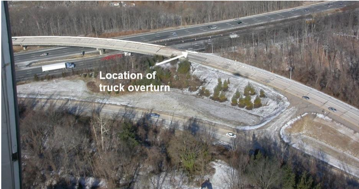
Figure 1. Aerial view of I-895 overpass, showing the accident location. (Courtesy of Maryland Transportation Authority Police Department)
