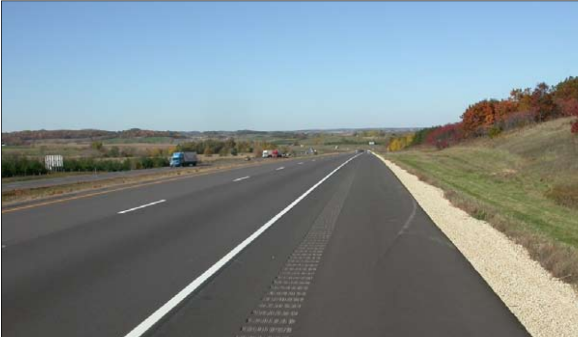
Figure 11. Rumble strips along the right shoulder of westbound I-94.
