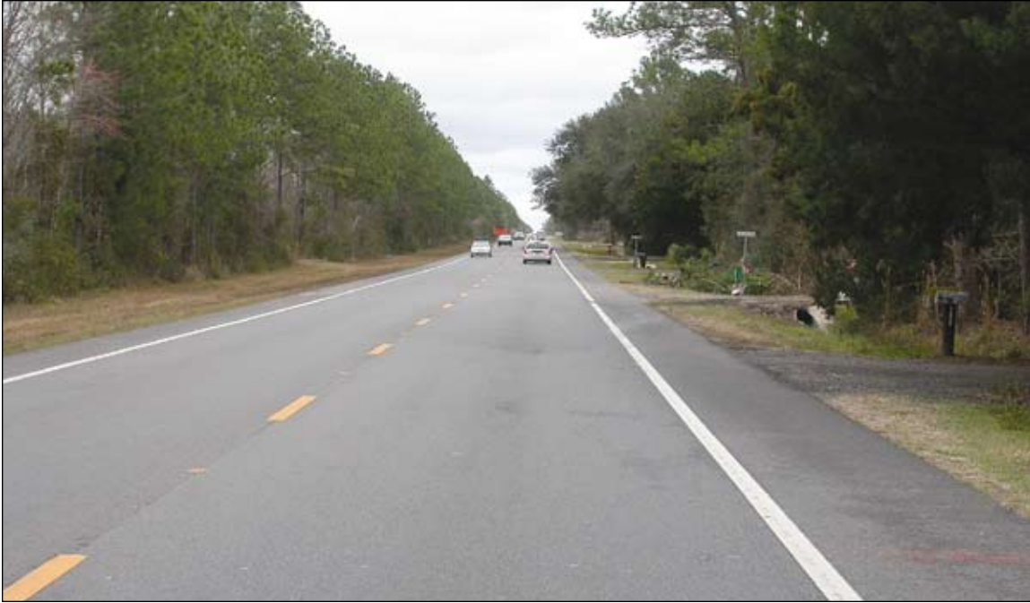
Figure 2. SR 121 approaching accident location.
