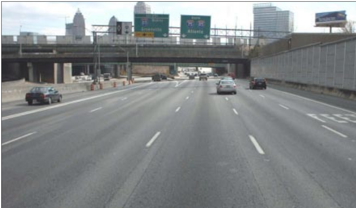
Figure 13. I-75 HOV lane diverging to the left in preparation for I-85 merge.
