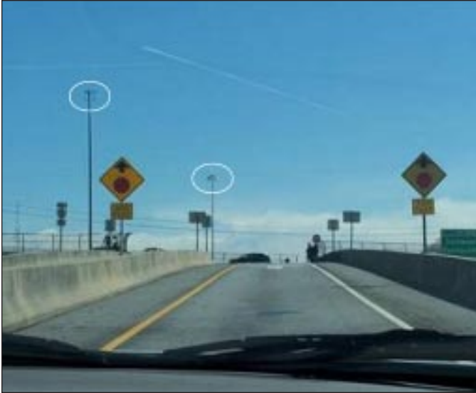
Figure 11. Exit ramp showing high-mast lighting (circled).
