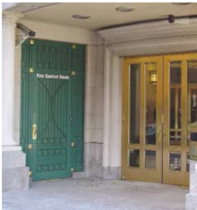
(Fig. 6.9) Fire command center next to main entrance. The sign on the room should be visible to responding firefighters.
