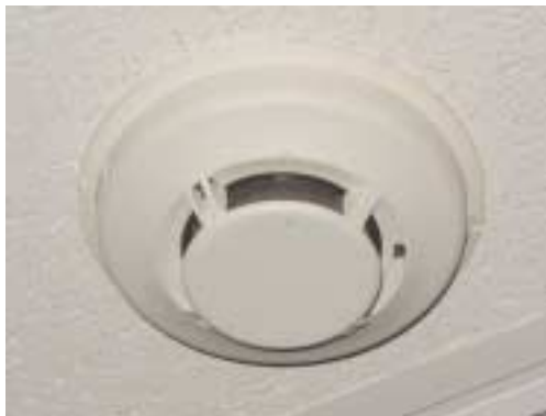
(Fig. 6.1a) Initiating device (smoke detector).
