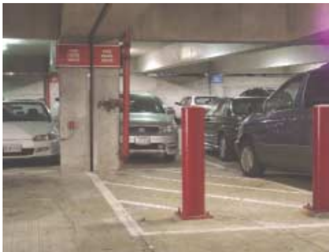
(Fig. 4.9) Bollards and striping to create an access path in a parking garage. Bright signs at the top of column help to locate the valve.
