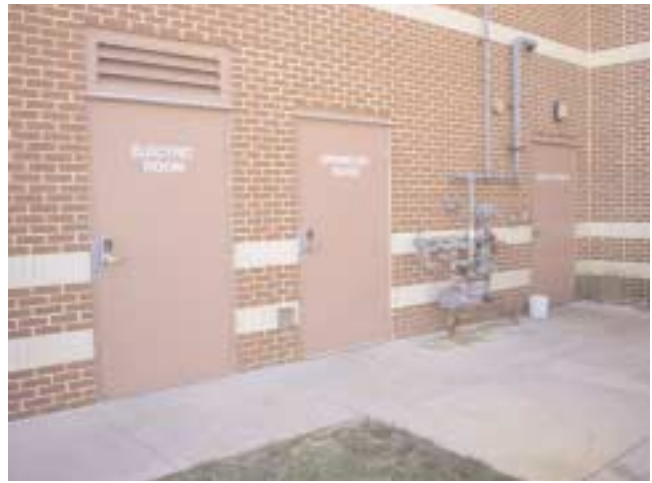
(Fig. 2.20) Rear doors of a shopping center labeled for rapid access: utility room, fire protection equipment room, and individual tenant space.
