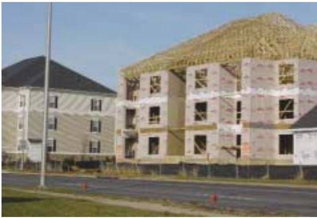
(Fig. 2.24) Building with wood truss construction. The adjacent finished building shows no indication from the exterior that wood trusses were used in its construction.
