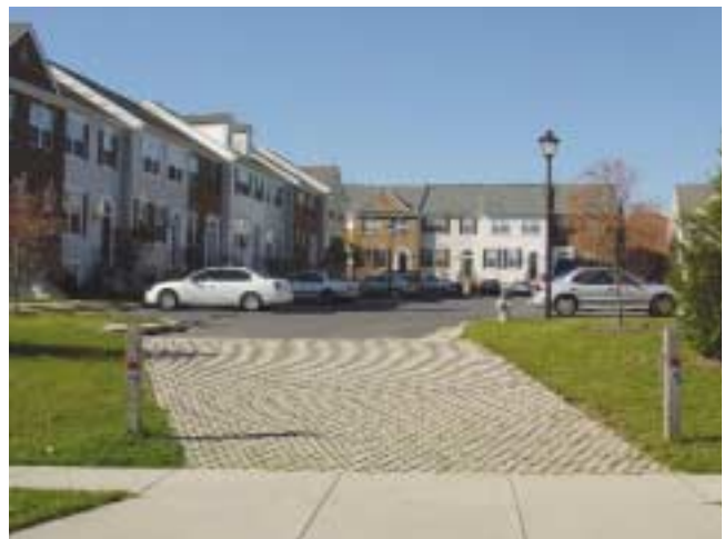
(Fig. 2.6) Paver blocks were chosen instead of paving for this access road. The aesthetic benefits are minimal, and the road cannot be plowed effectively.
