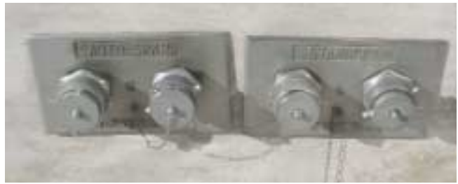
(Fig. 5.2) Separate sprinkler and standpipe connections (threaded types). To feed both systems, at least one hose line must be connected to each of the two FDCs.
