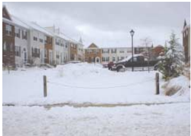
(Fig. 2.7) The same paver block access lane as shown in Figure 2.6, but covered with snow. Access is blocked by a mound of snow plowed from the adjacent parking lot.
