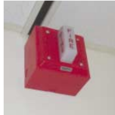
(Fig. 6.1c) Notification device (horn/strobe).
