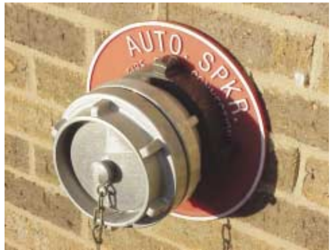
(Fig. 5.4) A quick-connect type of FDC.
