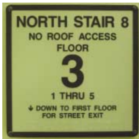
(Fig. 2.22) Stairway ID sign.
