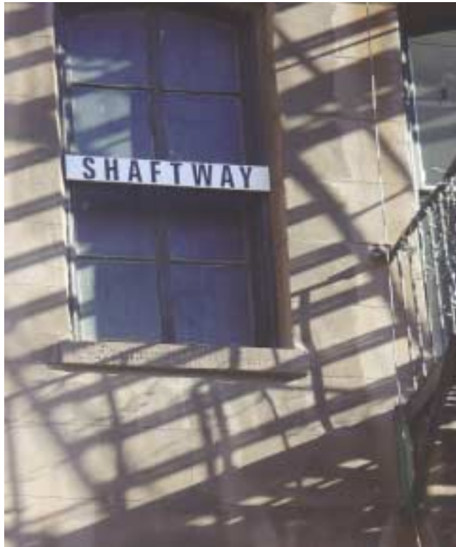
(Fig. 2.26) Exterior shaftway marking.
