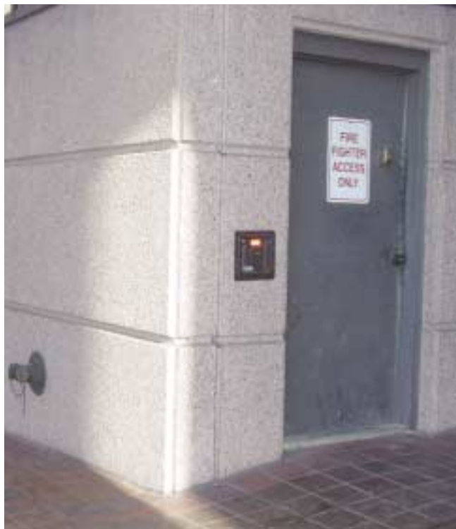
(Fig. 2.18) Key box adjacent to fire command center. These boxes are often provided at main building entry doors. Note the fire department connection on the left.
