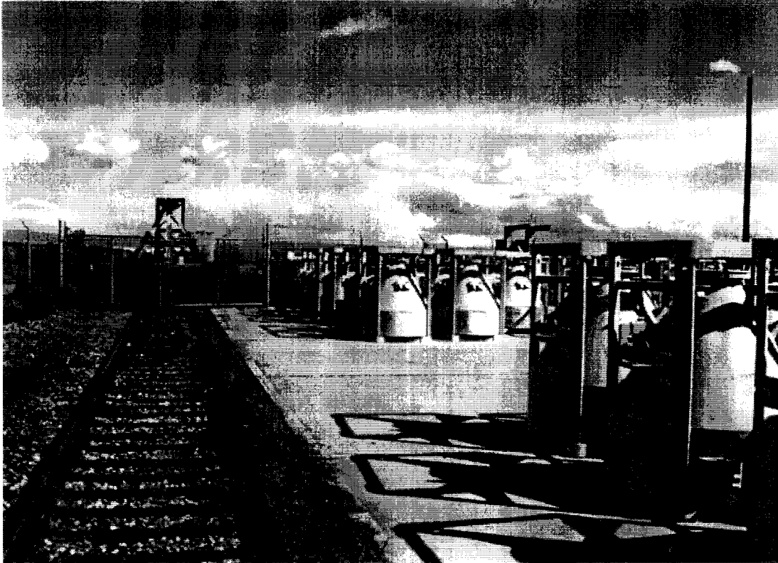
Figure 3-9 UO_3 T-Hoppers at Hanford Rail Spur, 200 West Area
