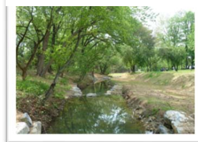
Watts Branch – After restoration
