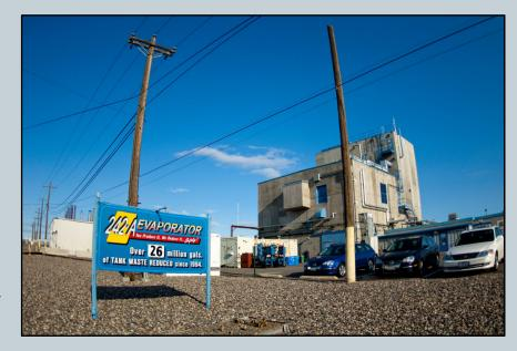
Why: The 242-A Evaporator reduces waste volume by removing water from the waste while letting dangerous constituents remain. The evaporator is essential for optimizing use of available tank space. The system is a single point failure; unplanned downtime will be a serious setback to future retrievals and transfers, and to feed availability for the Waste Treatment Plant.
