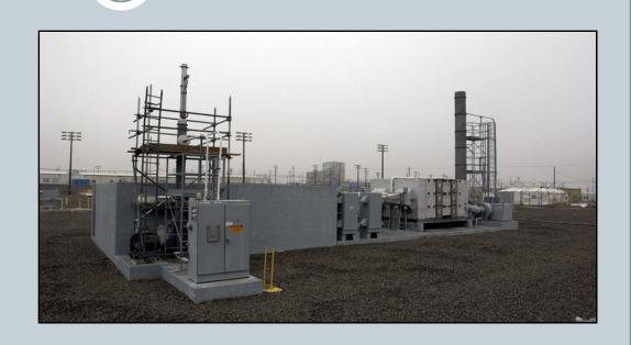
Why: Ventilation prevents buildup of flammable and corrosive gases in the tanks. Existing ventilation systems are unreliable and costly to maintain. New systems will simplify operations and prepare for waste transfer to the Waste Treatment Plant.
