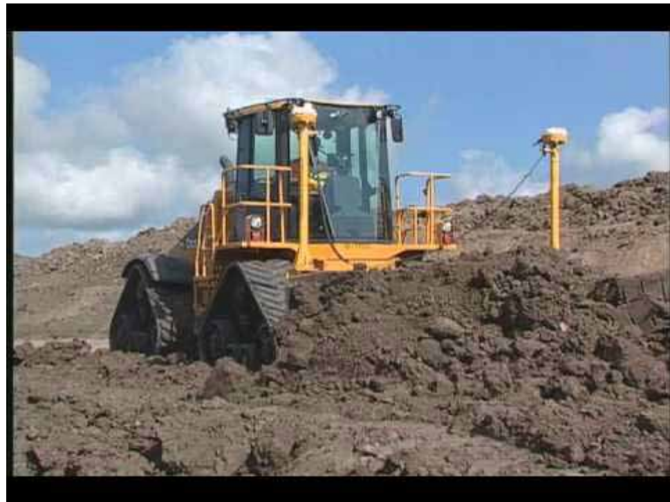
Soil Distribution over Site in Preparation for Backfill and Compaction
