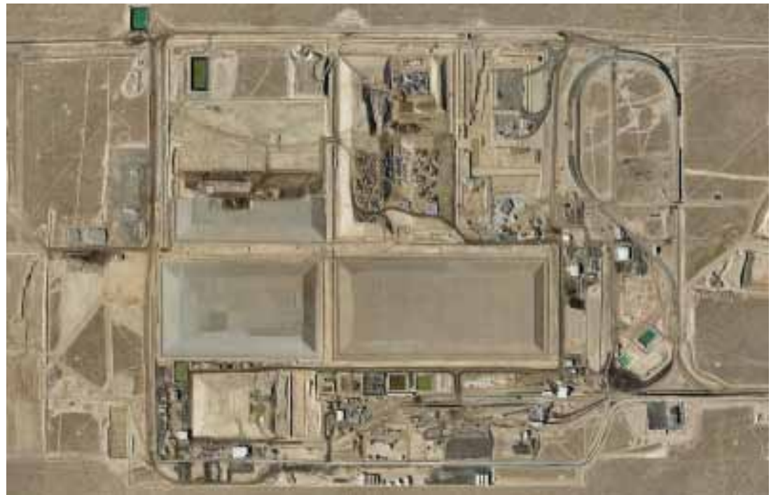
Energy Solutions Clive Utah Facility ( http://www.energysolutions.com )
