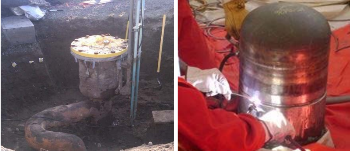
Figure 3-1. Excavated and Capped Cleanout Box
