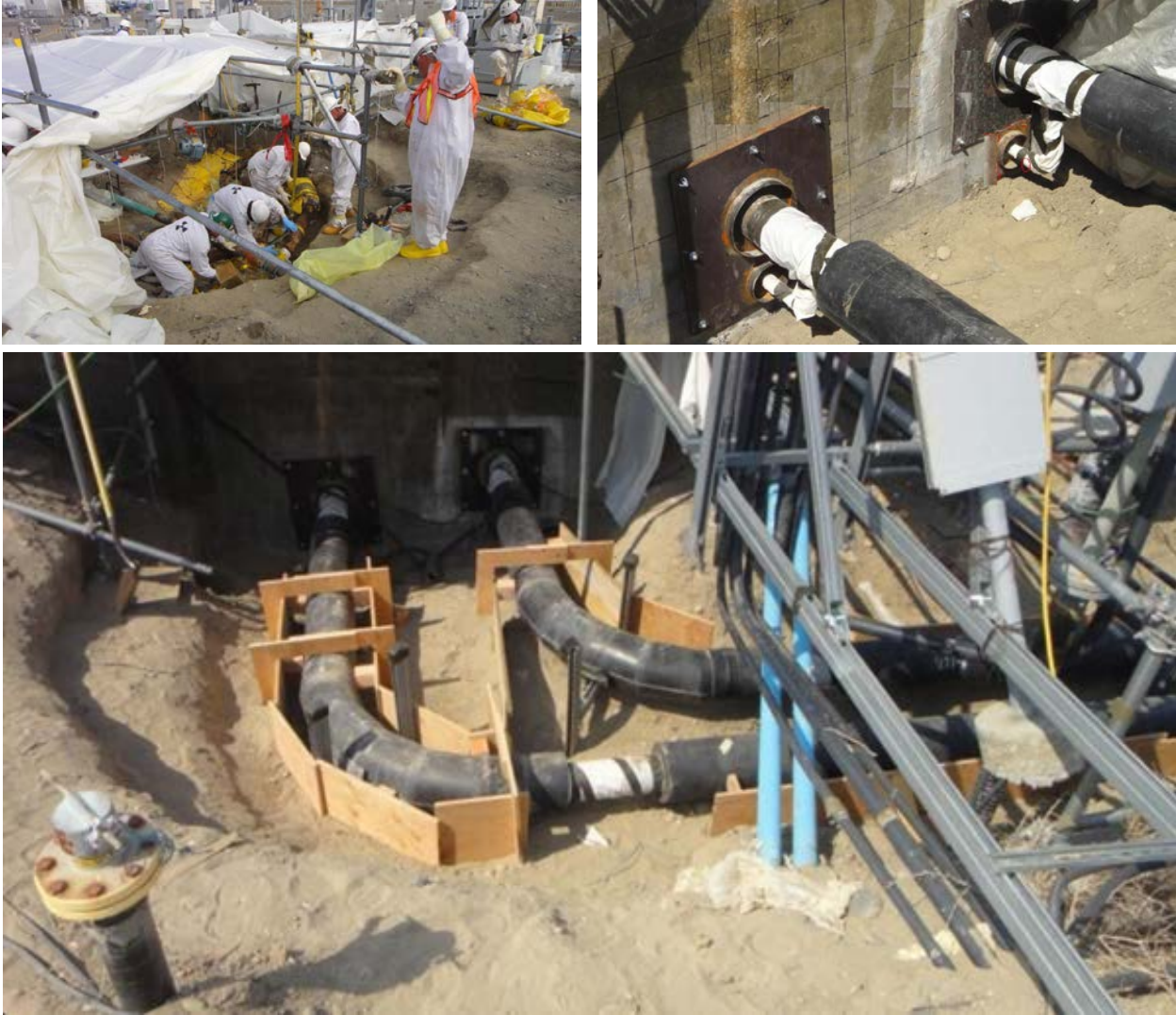
Figure 3-4. SY Farm Removal and Installation of Transfer Line Piping
