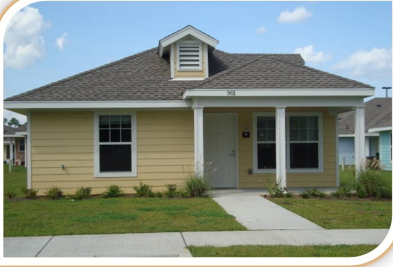
Gulf Coast Recovery Project—Bay Pines Apartment Typical Unit Jackson, Mississippi
