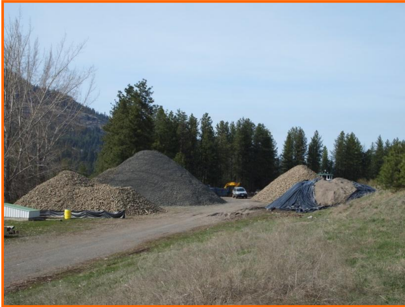
Rock storage on the opposite side of the Columbia River
