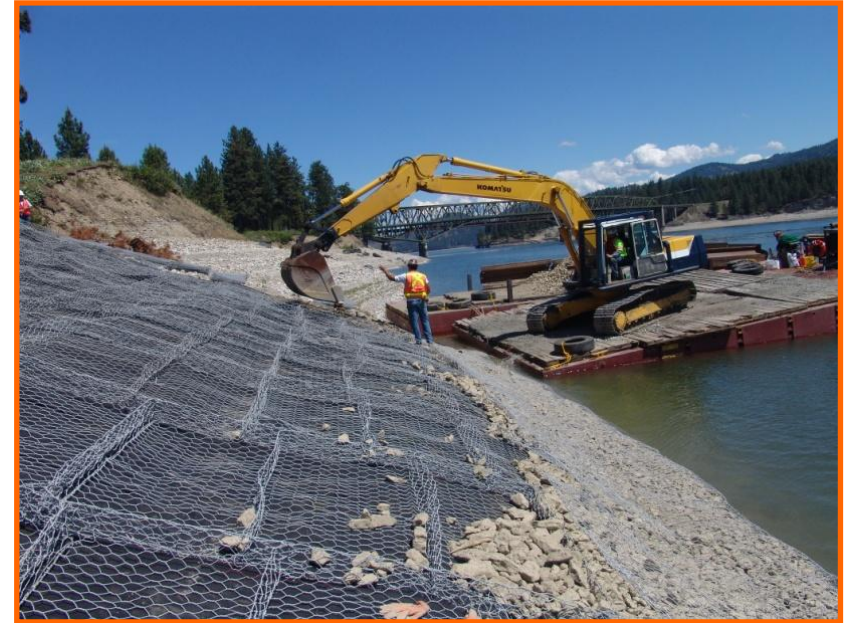
Installation of Reno mats using barge and track hoe
