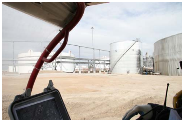
Figure 5.2-3: NIST staff collecting measurement data while driving around the perimeter of the facility among the large storage tanks.
