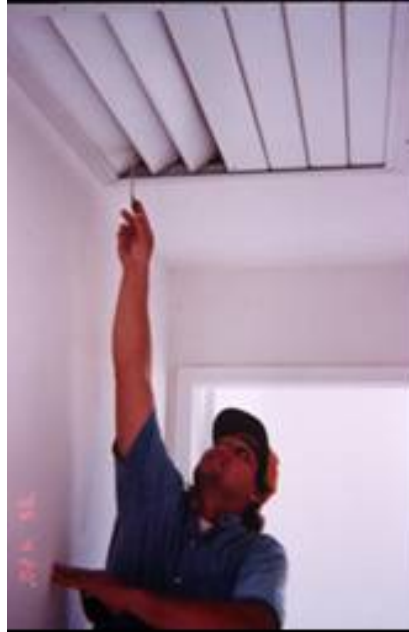
Figure 33. First WH fan installed showing operable louvers that open during operation
