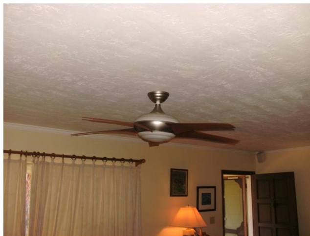
Figure 43. During the home remodel in 1998, high-efficiency ceiling fans were installed throughout the house to help shorten the A/C season (number of weeks A/C was necessary for comfort).
