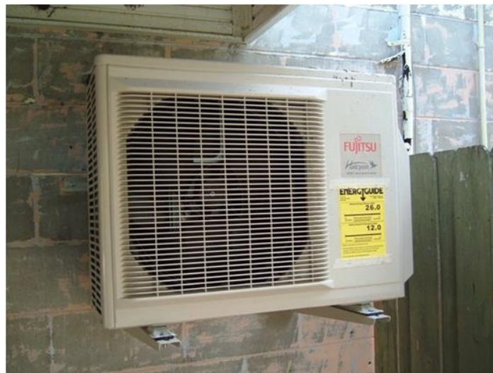
Figure 69. Outdoor unit of Fujitsu 9RLS mini-split heat pump as it appeared during the installation of the wall insulation retrofit. The outdoor unit is located outside the west garage.
