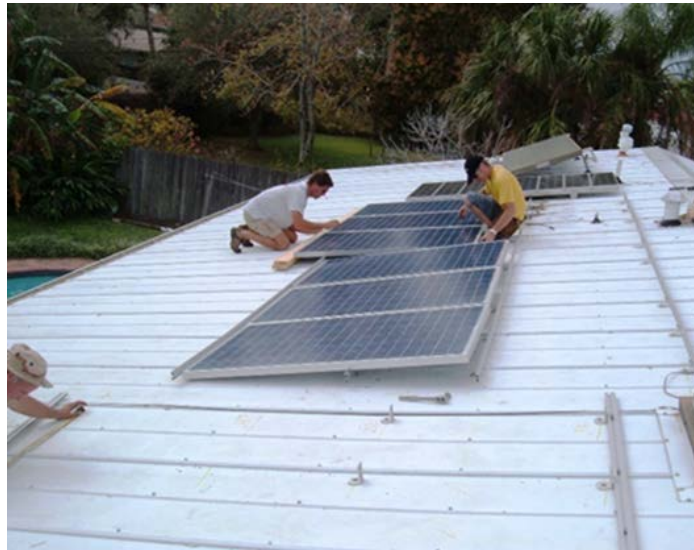
Figure 73. Installation of 4.1-kW PV system in February 2009
