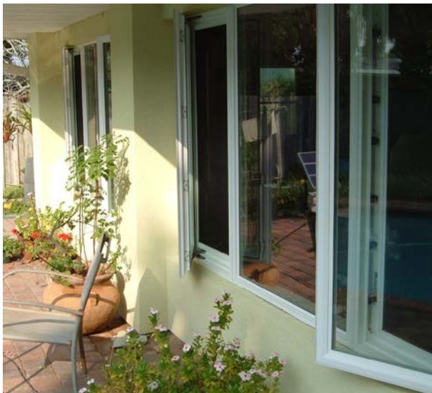
Figure 63. New high-efficiency solar control low-e windows on the south side of the home installed in August 2010. These casements open fully for ventilation.
