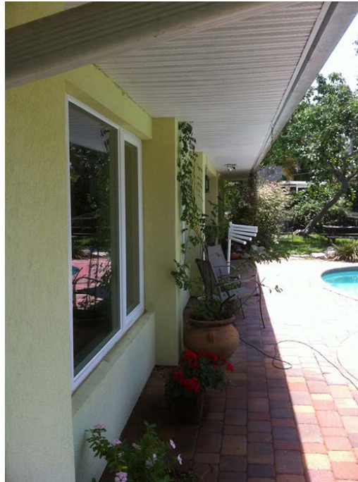
Figure 54. Three-foot overhang on the south face of the home and resulting shading pattern shown at noon on June 10, 2011. Note that the windows, walls, and foundation are fully shaded.
