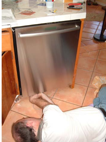
Figure 61. Installation of new ENERGY STAR dishwasher
