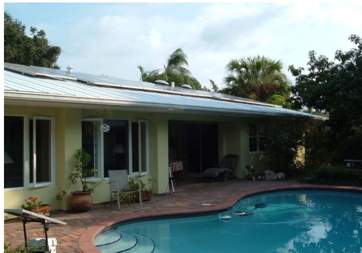
Figure 67. PV-powered pool pump in operation with the automatic pool cleaner operating during daytime. This retrofit saved at least 2000 kWh/year.
