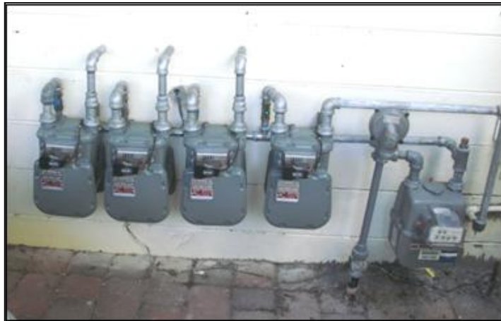
Figure 6. Multiple pulse initiation gas meters to measure gas end use
