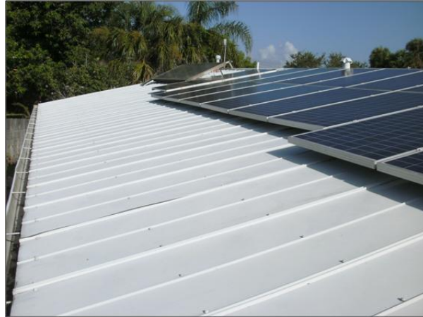
Figure 42. White metal roof after 12 years of weathering on the south exposure. The 5-vee metal panels have maintained their reflectance. PV modules are seen in the image with the solar water heater at the far end.
