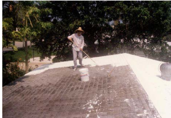
Figure 40. A highly reflective elastomeric coating was applied over shingles in an experiment in July 1992 (a practice that is no longer recommended because of moisture-related problems)
