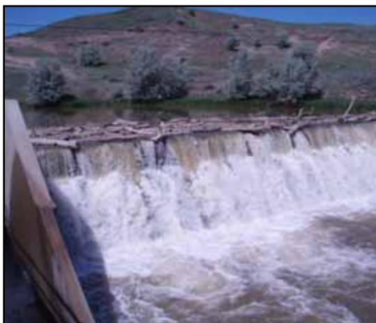
Figure 1.4: Paradise Valley Irrigation District Diversion Dam.
