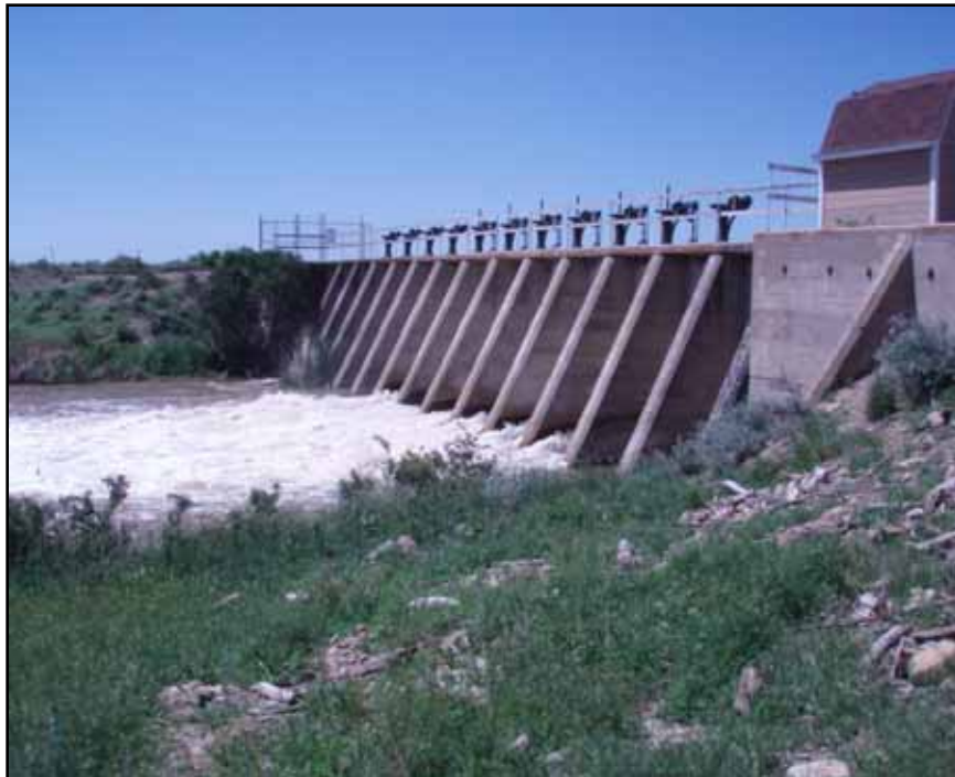
Figure 2.4: Dodson South Canal headworks.
