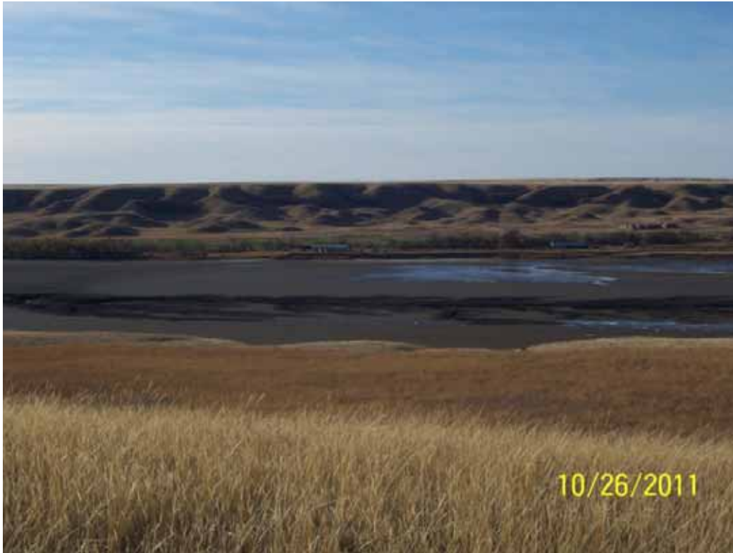
Figure 5.10: Frenchman Reservoir dewatered during 2011 construction activities.
