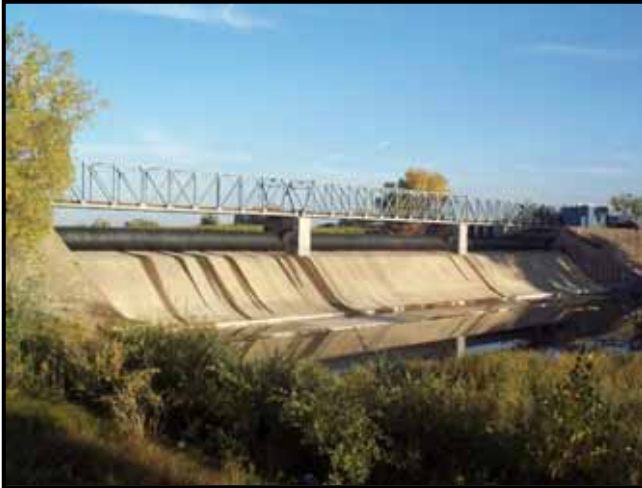
Figure 3.1: Dodson Diversion Dam.
