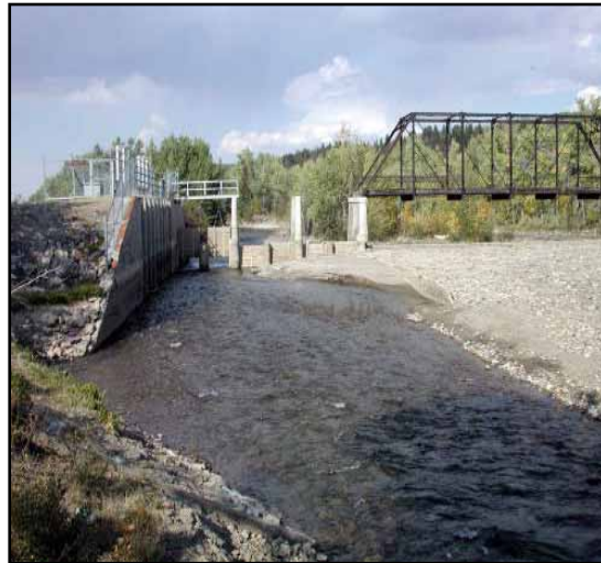
Figure 1.7: St. Mary Diversion Dam at low flow.
