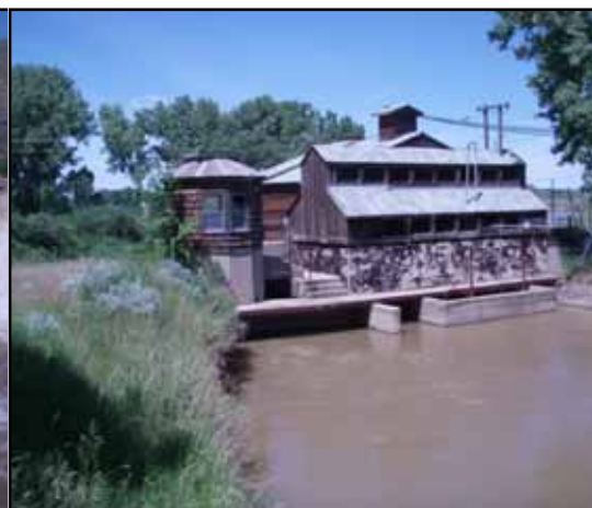
Figure 1.5: Harlem Irrigation District main pump station.
