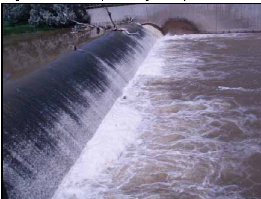
Figure 2.12: Fort Belknap Indian Irrigation Project Diversion Dam.
