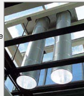
Example of Solatube daylighting system for commercial use.
