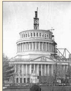
Construction of the new cast-iron dome was well under way in 1861 (left).
