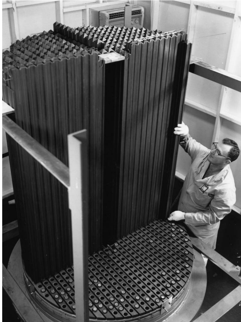
Fig. 23. Graphite core of the MSRE.
