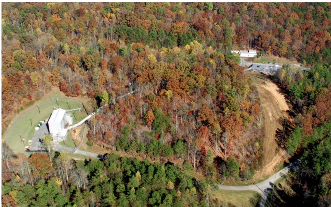
Fig. 28. The DOSAR facility. The HPRR is at lower left, and the control and laboratory building is at upper right. (ORNL Photo 3816-99)
