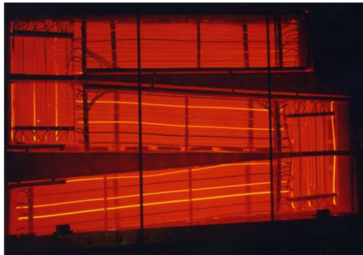
Fig. 26. MSRE air-cooled radiator with its door open.
