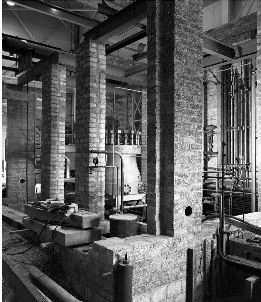
Fig. 11. The HRE pressure vessel during construction. (ORNL Photo 8614)
