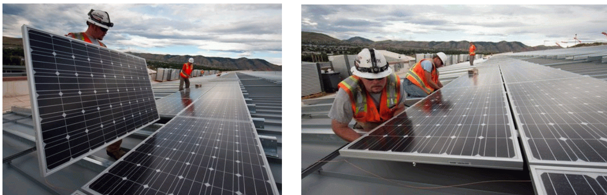
Figure I-4 Installation of a nonresidential CSPV system
