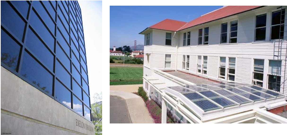
Figure I-2 Building integrated CSPV
