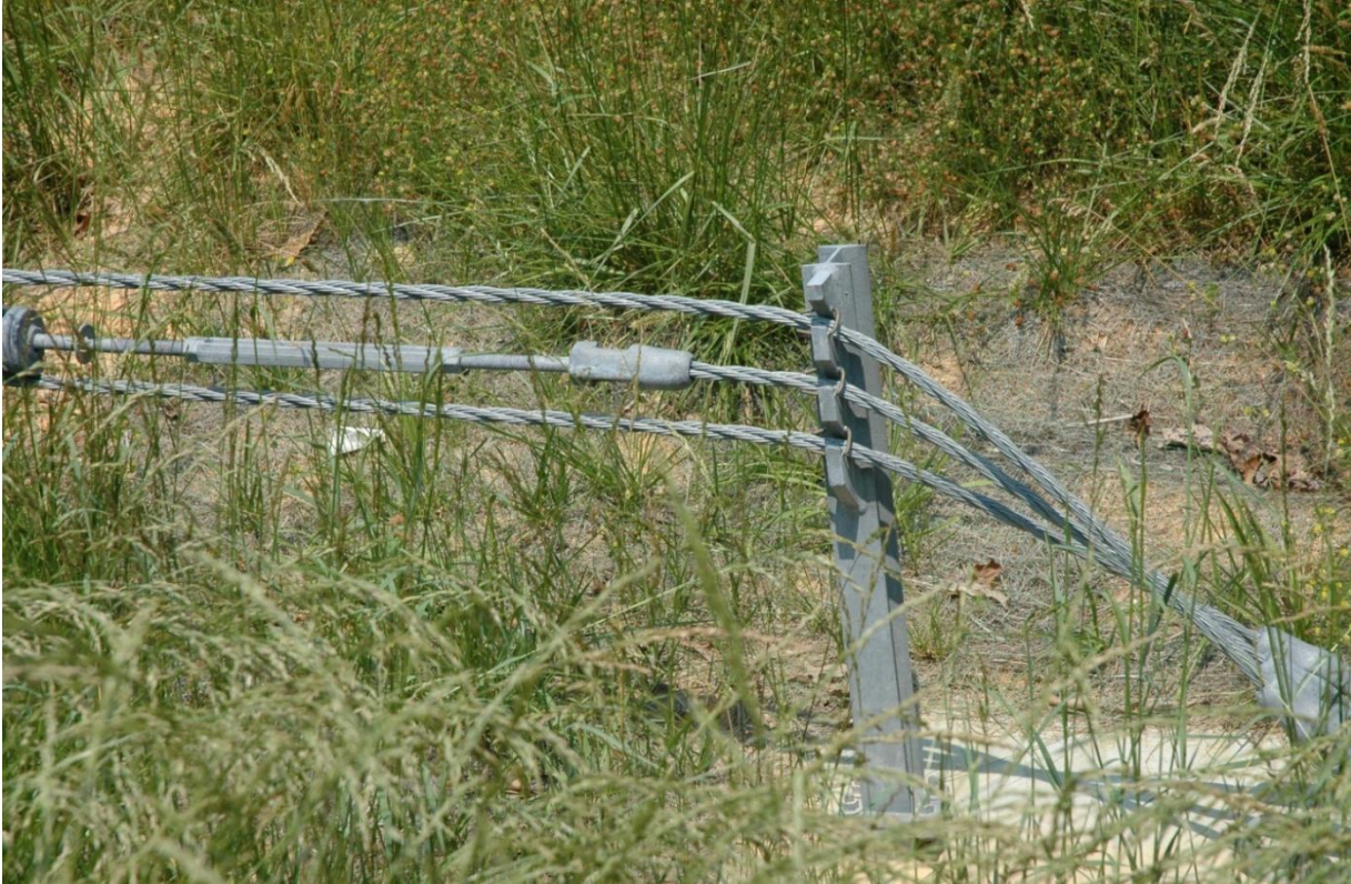
Figure 11. Three-strand cable barrier near accident site.
