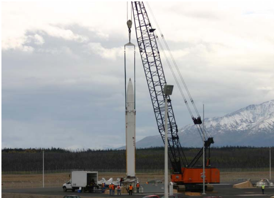
PHOTO CAPTION: The second interceptor missile designed to intercept and destroy a long-range ballistic missile is emplaced into its underground silo at Ft. Greely, Alaska.
