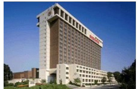
Sheraton National Hotel 900 S. Orme Street Arlington, VA
