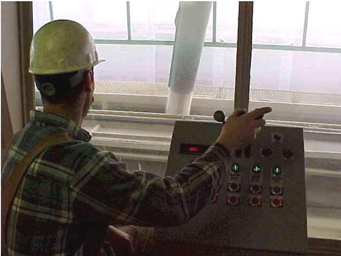
Figure 7.8. Environmentally controlled operator's booth near loadout area.
