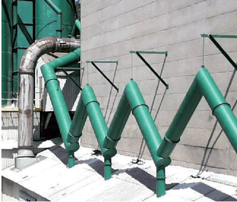
Figure 1.10. Sawtooth design of a low-velocity system with a dropout duct back into the process at the base of each leg.
