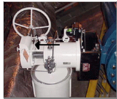
Handwheel Disengaged
