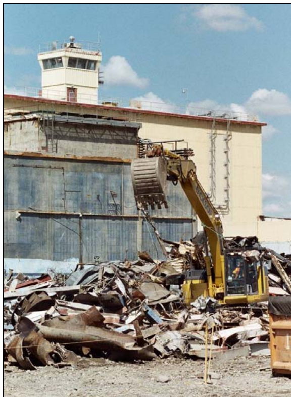
Demolishing facilities at the N Reactor
