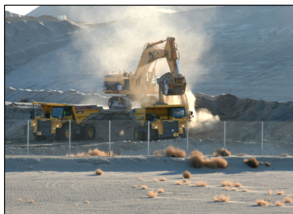
Excavating a new disposal cell at the Environmental Restoration Disposal Facility
