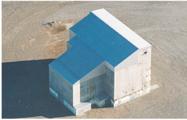
Reactor Safe Storage and D&D of Surplus Facilities
