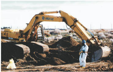
Remove and Dispose of Contaminated Soils
