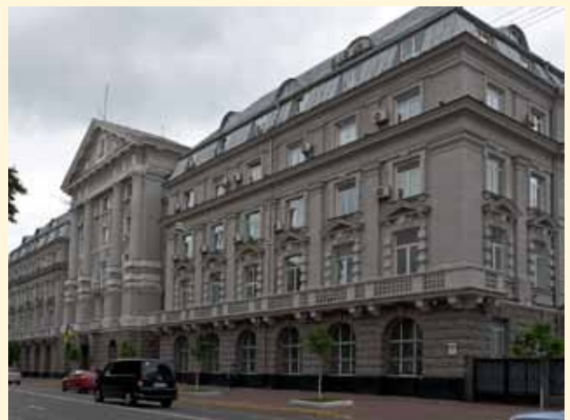
Building of SBU (Security Service of Ukraine)
