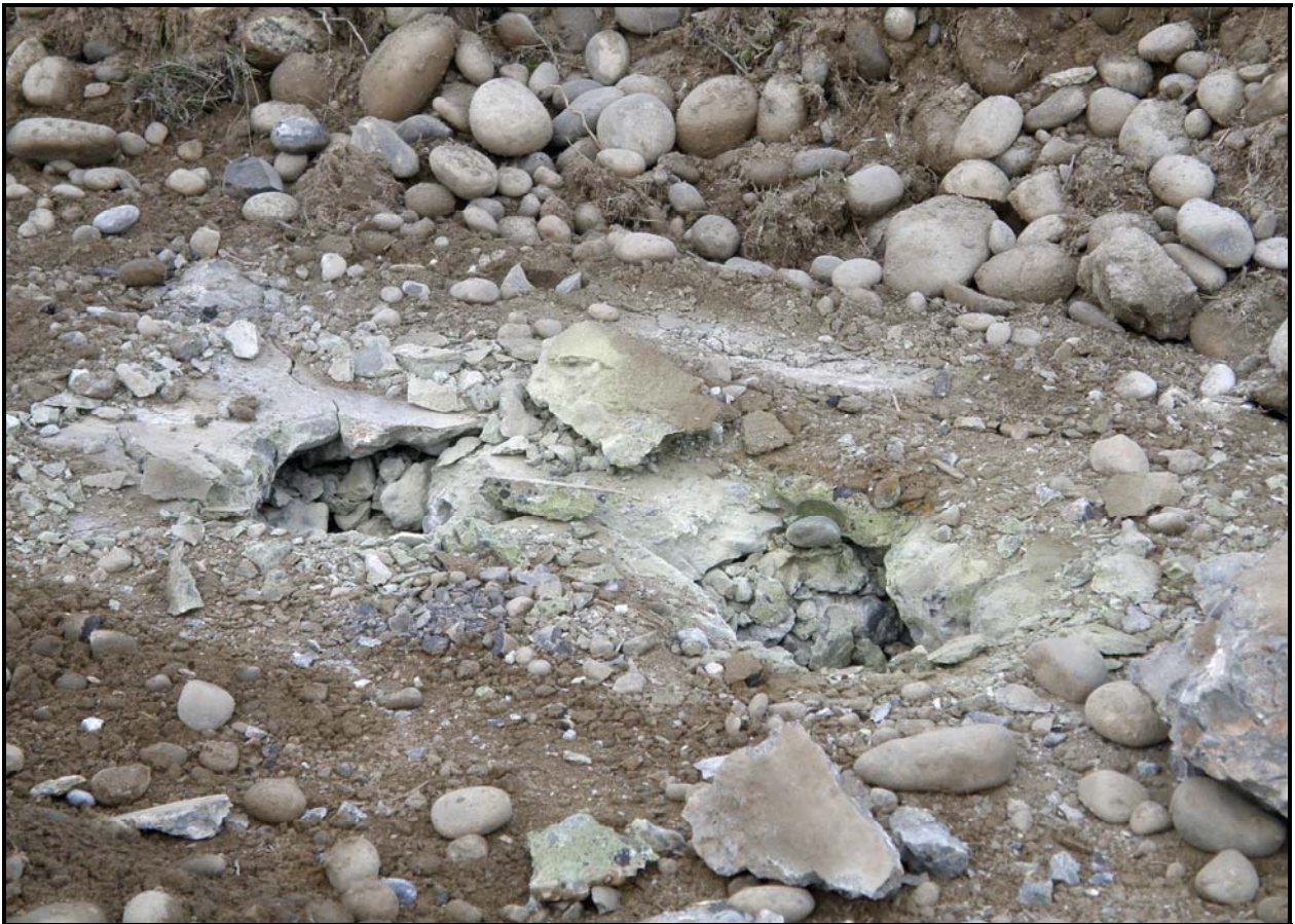
Stained concrete was discovered at 100-F-57 last month during remediation activities at 100-F Area. Sampling confirmed the presence of hexavalent chromium in the area. (Photo 6)
