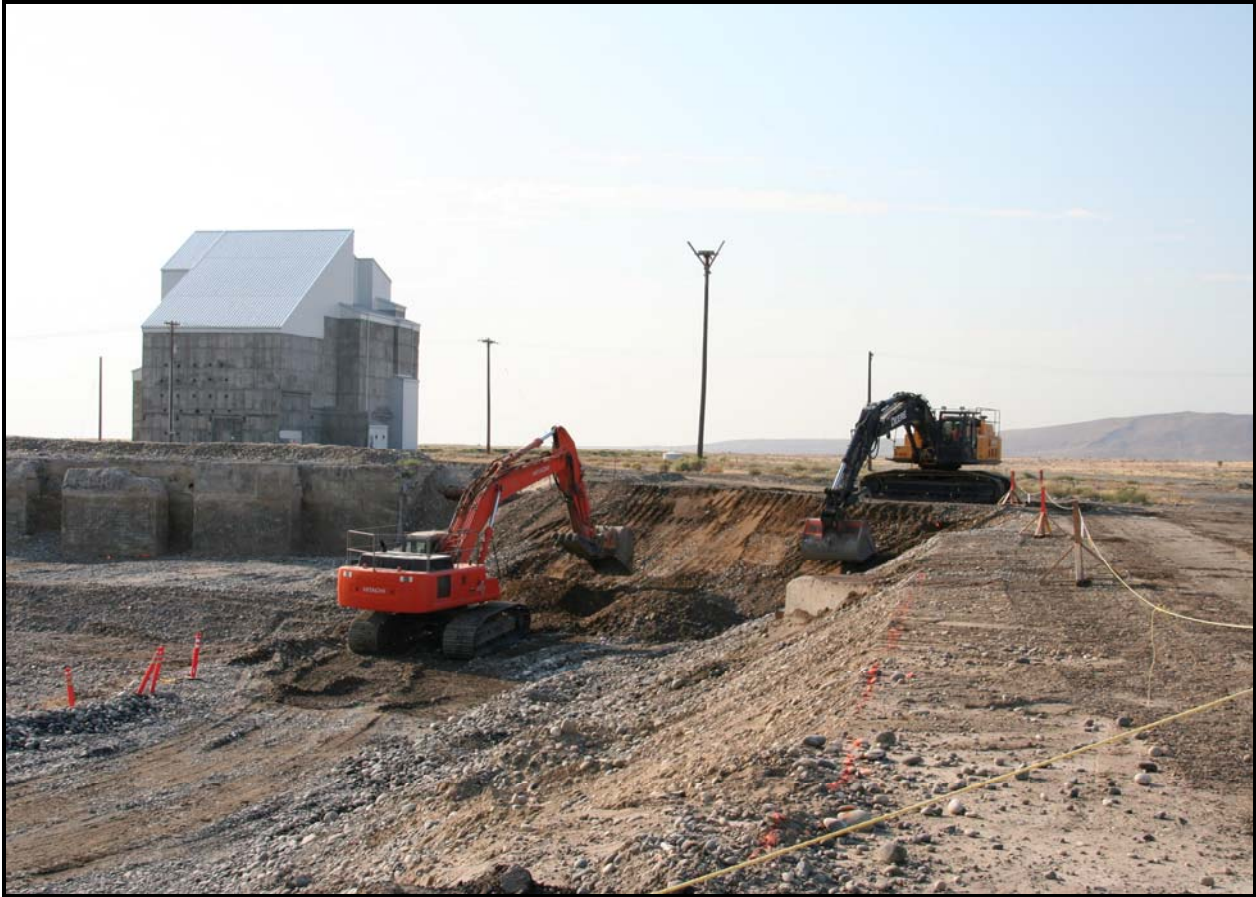
F Reactor operated from 1945 to 1965 as one of Hanford's nine surplus plutonium production reactors for the nation's nuclear weapons program. The reactor was cocooned in 2003. During reactor construction and operations, waste was disposed in unlined pits and trenches throughout the site. (Photo 5)
