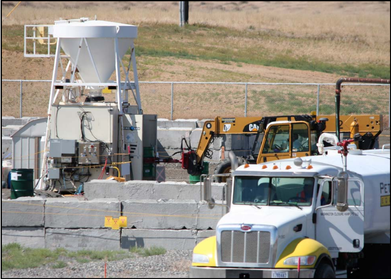
A drum is placed inside a drum punch during trench remediation activities at the 618-10 Burial Ground. (Photo 5)
