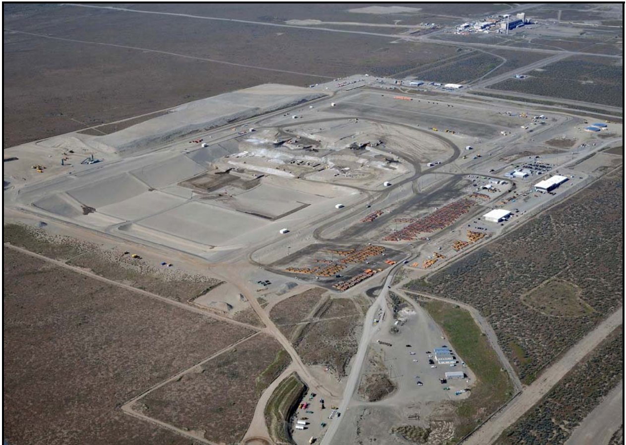
An aerial photo shows the Environmental Restoration Disposal Facility from the northeast corner of the facility. (Photo 1)
