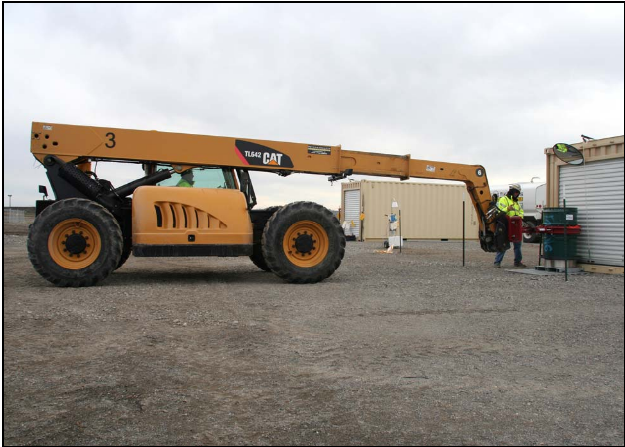
A telehandler operator conducts mockup exercises at the 618-10 Burial Ground. (Photo 7)
