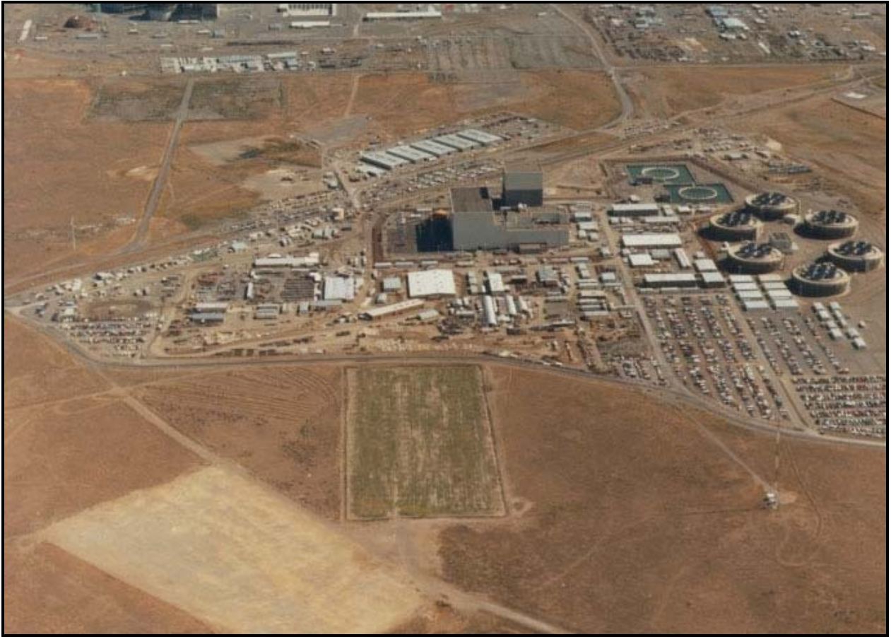
The 618-11 Burial Ground is located next to the Energy Northwest's Columbia Generation Station, an operating commercial nuclear power plant. (Photo 7)
