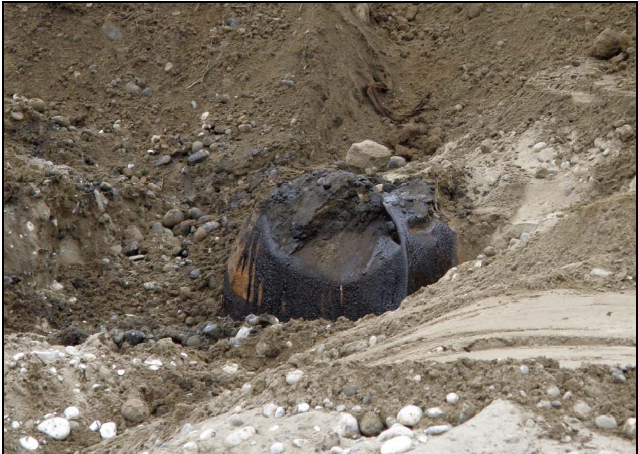
A storage tank was discovered at the site containing an old maintenance garage lube pit foundation. Sampling of the soil around the tank was conducted. (Photo 7)
