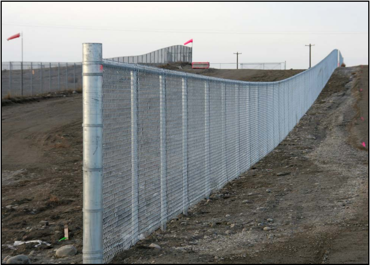
White Shield/Apollo installed new perimeter fencing at the 618-10 Burial Ground. (Photo 6)
