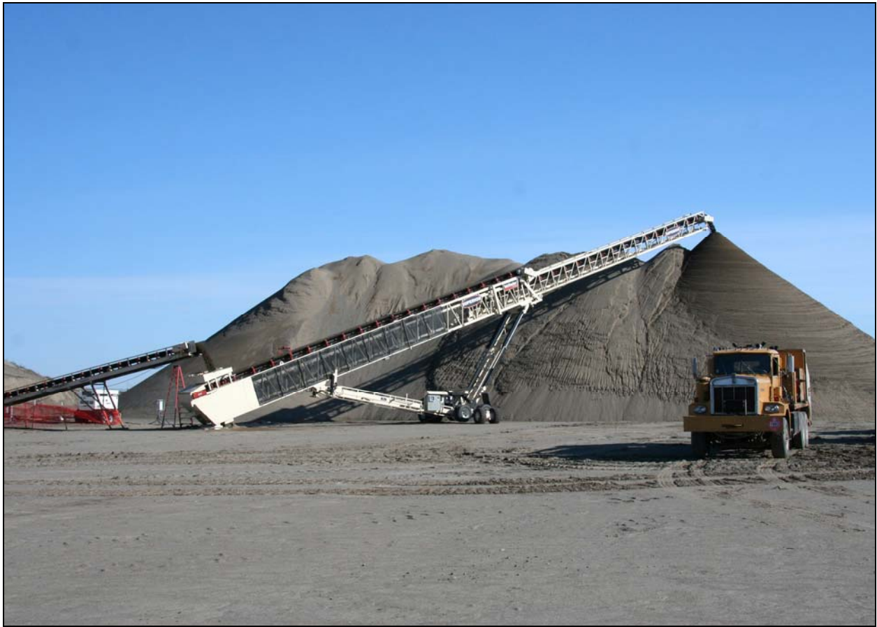
Sand for ERDF's new batch plant continues to be stockpiled. The batch plant will be used to manufacture grout for disposal operations. (Photo 4)
