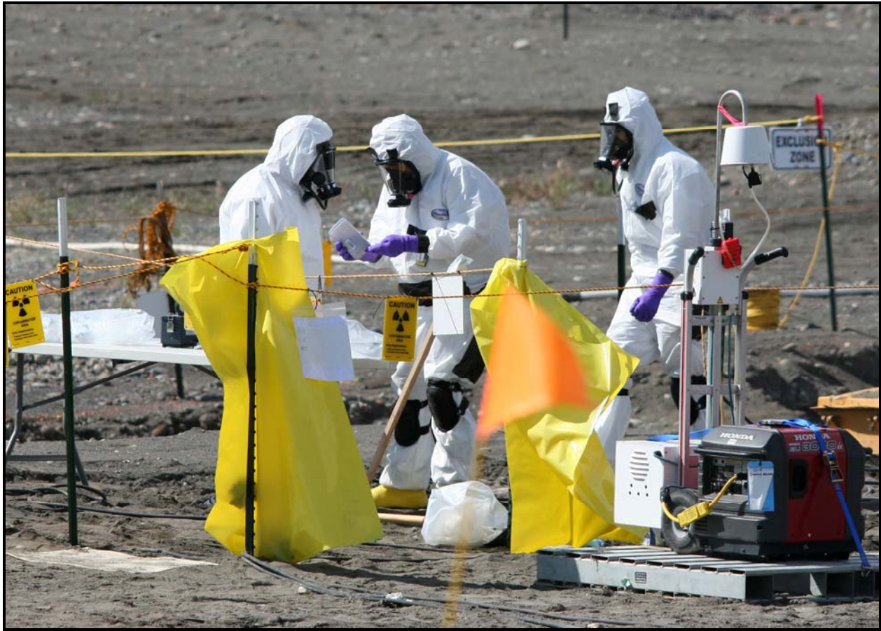
Samples are collected during trench excavation at the 618-10 Burial Ground. (Photo 9)
