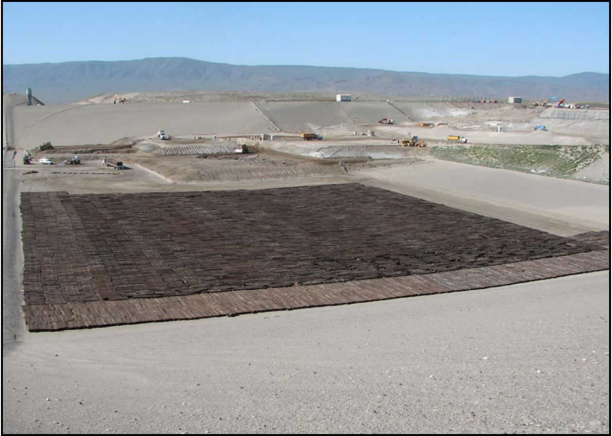
Railroad ties from the Hanford Site continue to be disposed in super cell 9. ERDF is expected to receive nearly 60,000 railroad ties. (Photo 2)
