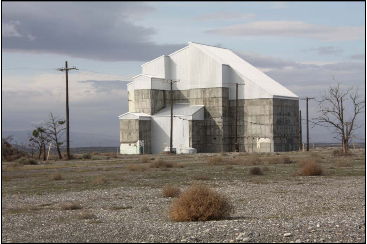
F Reactor operated from 1945 to 1965 and was placed in interim safe storage in 2003.
