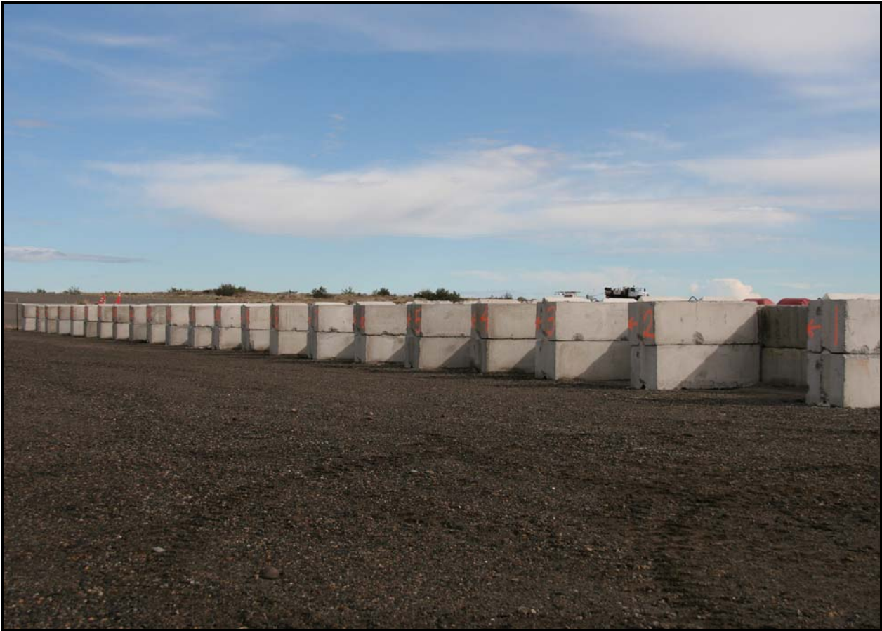
The drum storage area has been set up in the staging area at the 618-10 Burial Ground.
