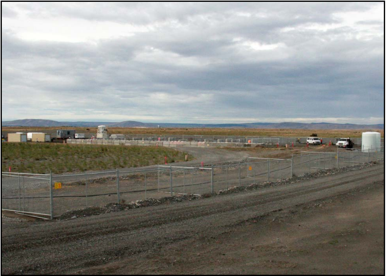
Work continues setting up the staging area at the 618-10 Burial Ground.
