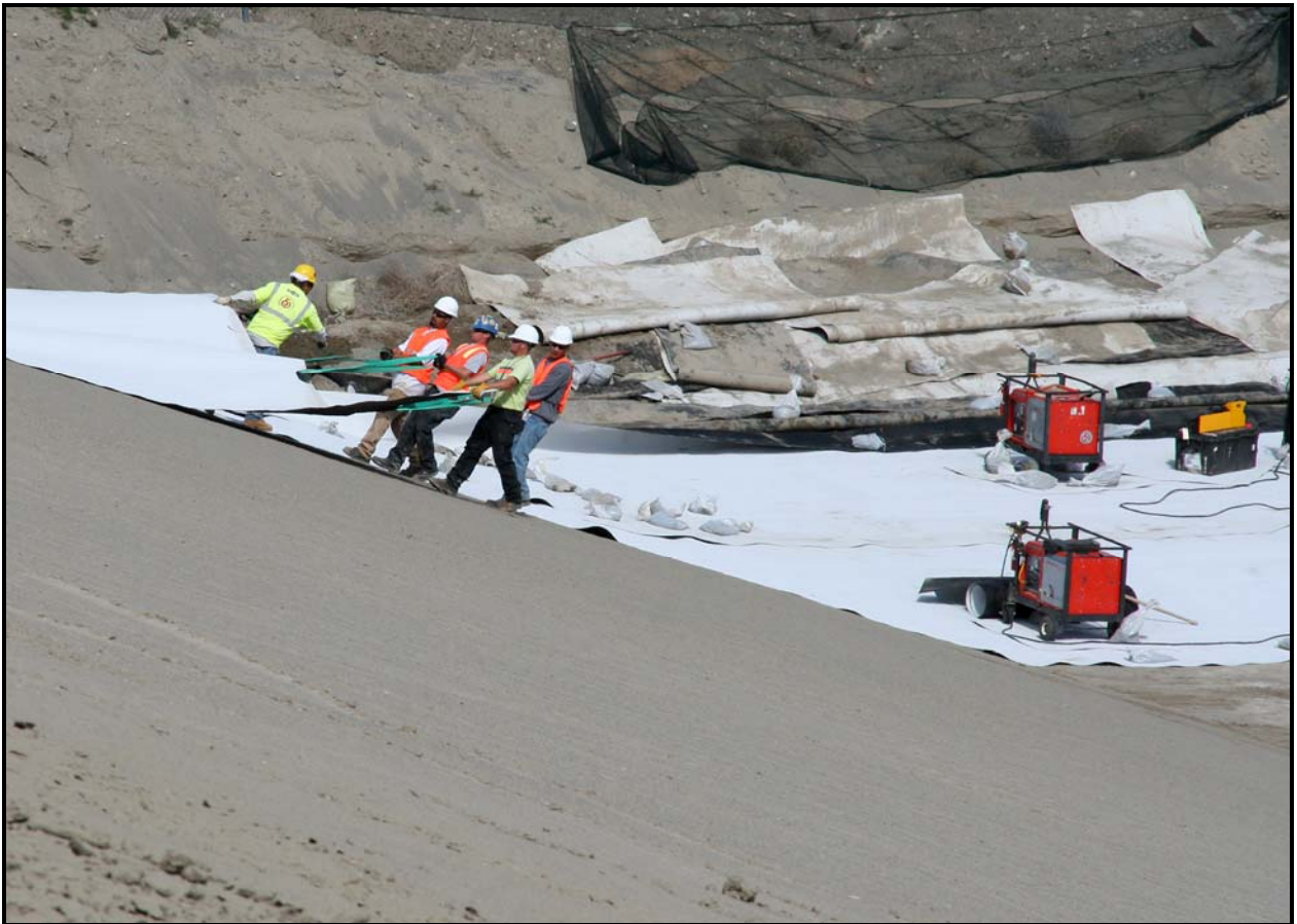
TradeWind Services/DelHur Industries personnel roll a section of 60-mil high-density polyethelene geomembrane liner down the slope of super cell 9 at the Environmental Restoration Disposal Facility.
