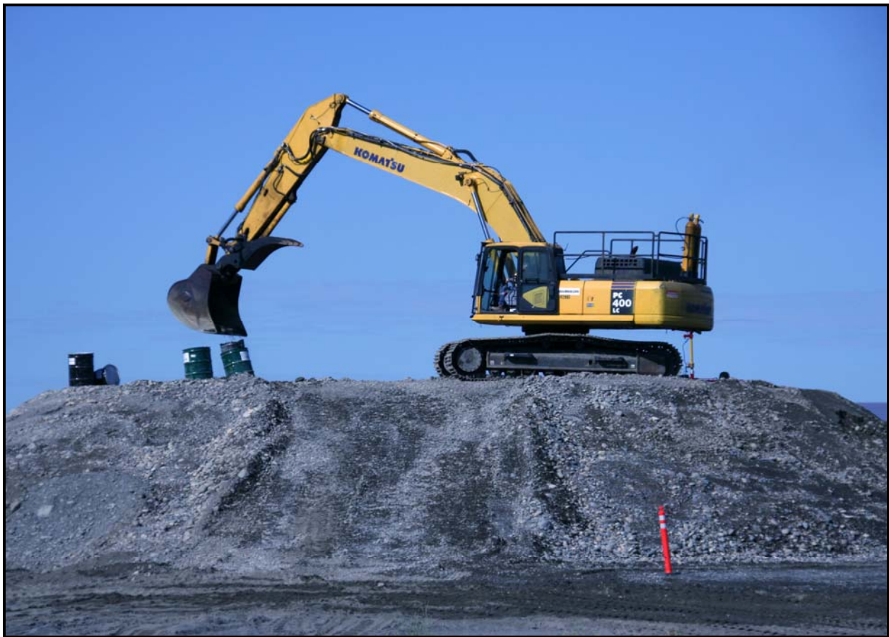
An excavator practices removing drums during a mock-up for intrusive characterization at the 618-10 Burial Ground.
