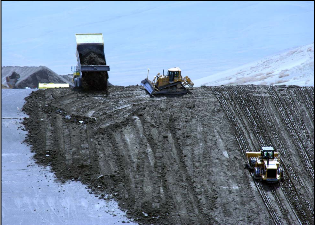
TradeWind Services/DelHur Industries personnel continue to place admix on the south slope of super cell 9 at the Environmental Restoration Disposal Facility.
