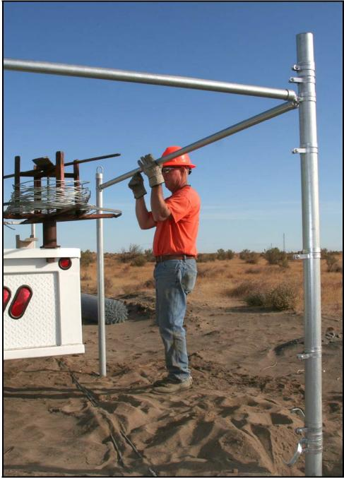
More than 8,700 feet of chain link fencing is being installed around the perimeter of the new Environmental Restoration Disposal Facility super cells 9 and 10.
