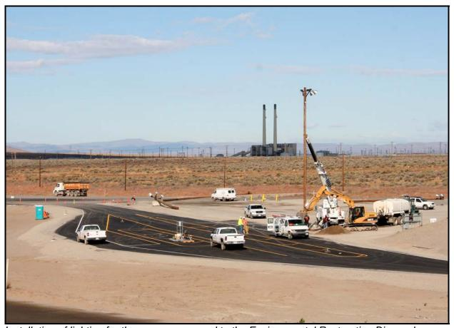
Installation of lighting for the new access road to the Environmental Restoration Disposal Facility is underway, and striping was completed.
