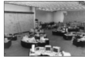
Under BPA's separated functions, transmission dispatchers can change generation levels in real time if necessary to avoid outages.
