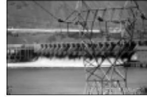
BPA has separated its transmission and power functions.
