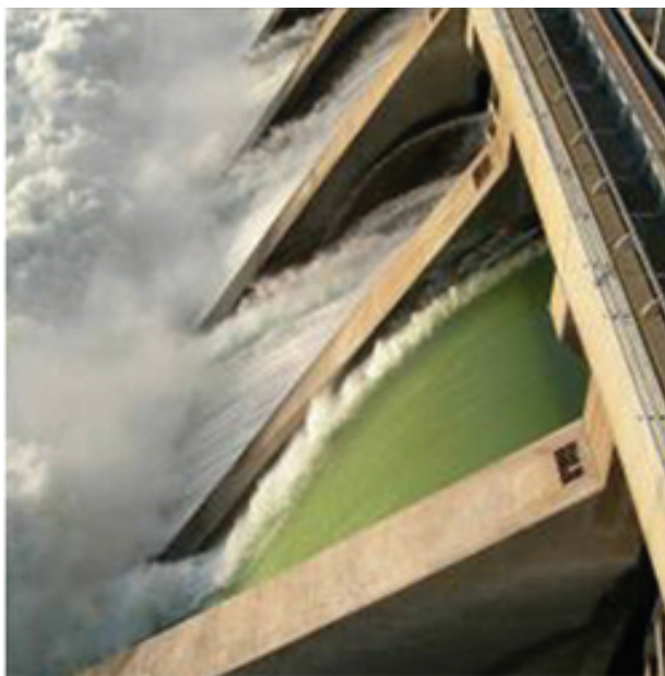
The smooth green water of a fish weir lets young salmon slide over a dam in the surface water they prefer. (U.S. Army Corps of Engineers photo)
