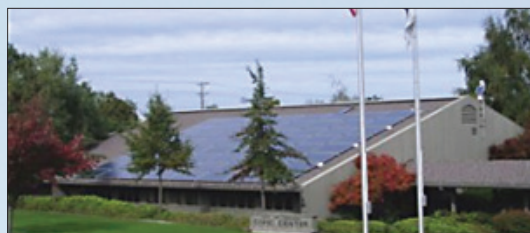
Solar units on the Ashland Police Station.
