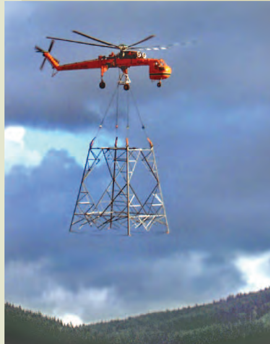
Flying towers by helicopter cuts construction impacts.
