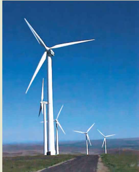
Stateline wind turbines on Vansycle Ridge on the Washington-Oregon border.
