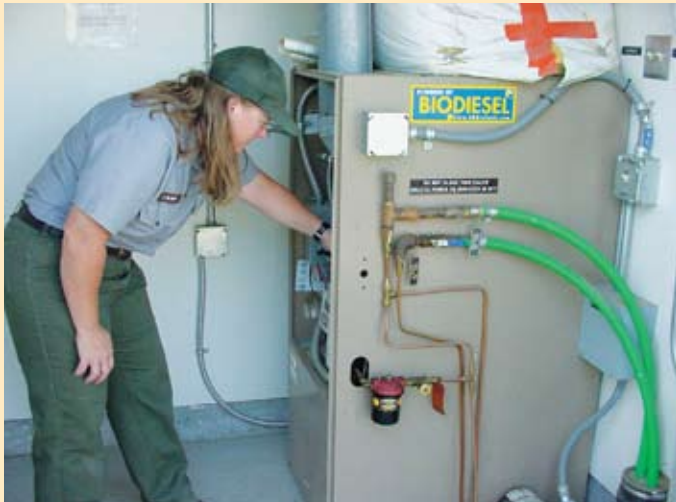
Maintenance Worker Diana Elder checks a biodiesel-powered furnace. The biodiesel blend helps Whitman Mission reduce nitrogen oxide and sulfur dioxide emissions.
