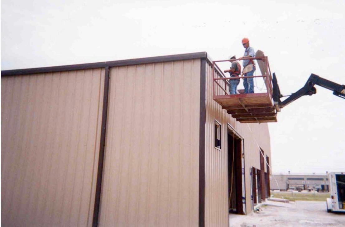
The same building is shown in the last phase of construction.
