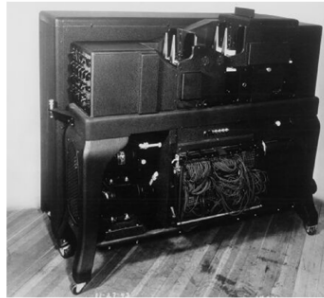
IBM Relay Calculator, 1944
