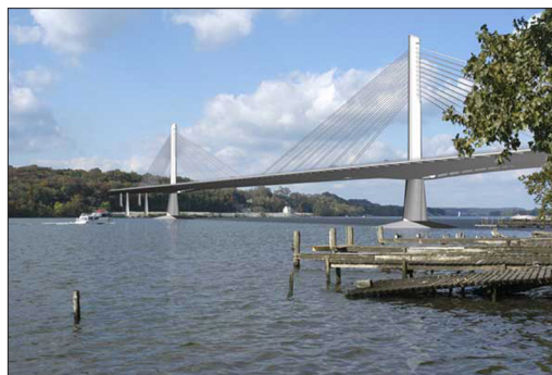
The boat dock depicted on the Kentucky shoreline indicates this section of the river is popular with recreational boaters, which is one reason for the wide distance between the bridge piers. (photo courtesy the Ohio River Bridges Project)
