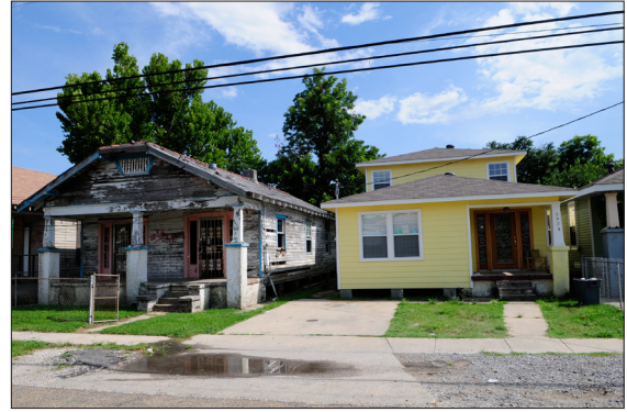
This photo, taken in New Orleans, LA, July 8, 2008, shows houses in the Jackson Barracks community of the 9th Ward, reflecting the pace of recovery, one house at a time. Barry Bahler/FEMA
